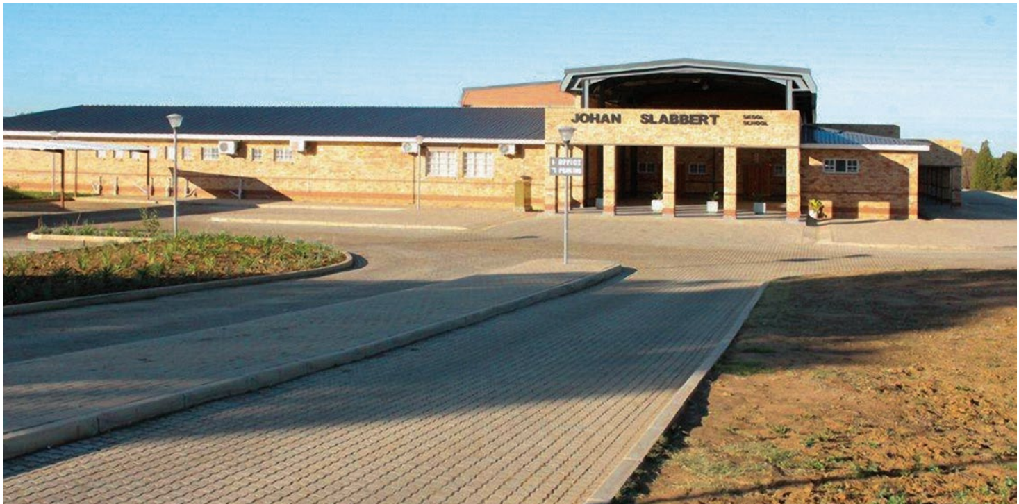
The Johan Slabbert Special School in Kroonstad was successfully delivered to the Department of Education in good time and is operational
